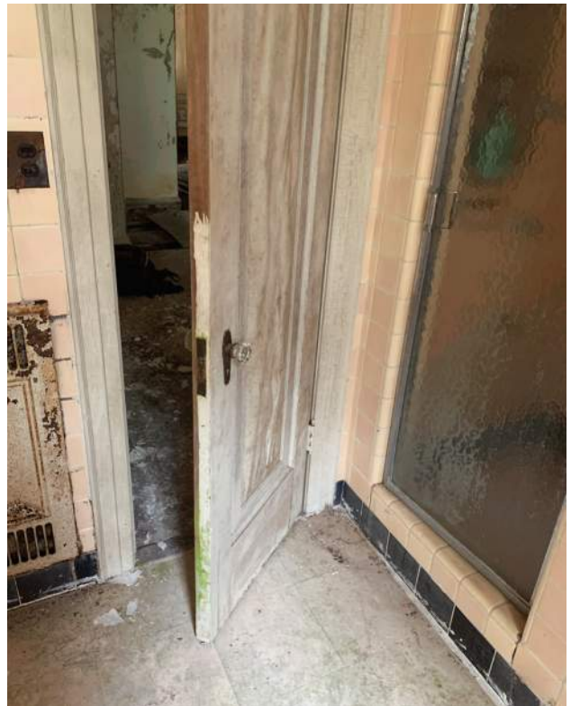
Shower Area of First Floor Level Bathroom
