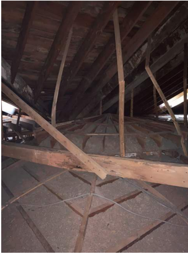
Attic Bracing Above Reception Room Dome
