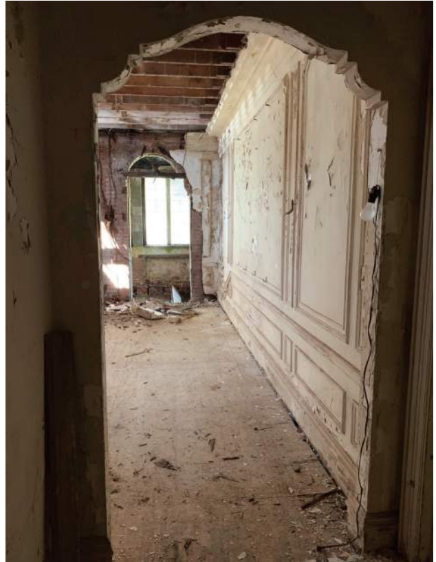
View Towards West Sunporch
