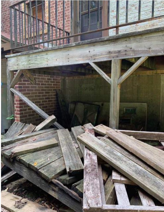
Wood Framed Platform on Rear of Building
