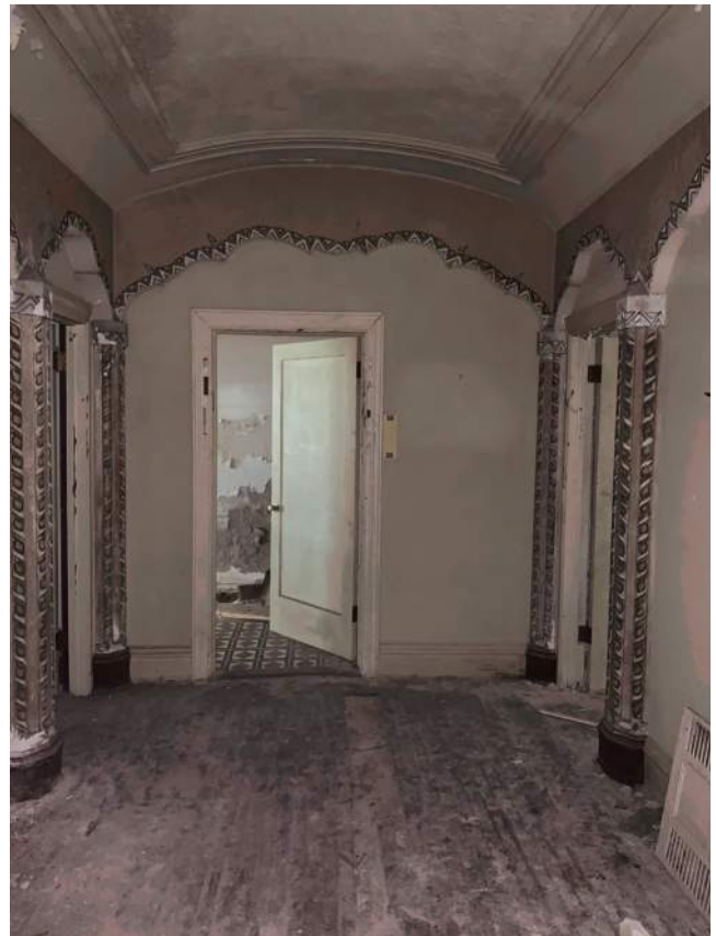
Lobby Looking North
