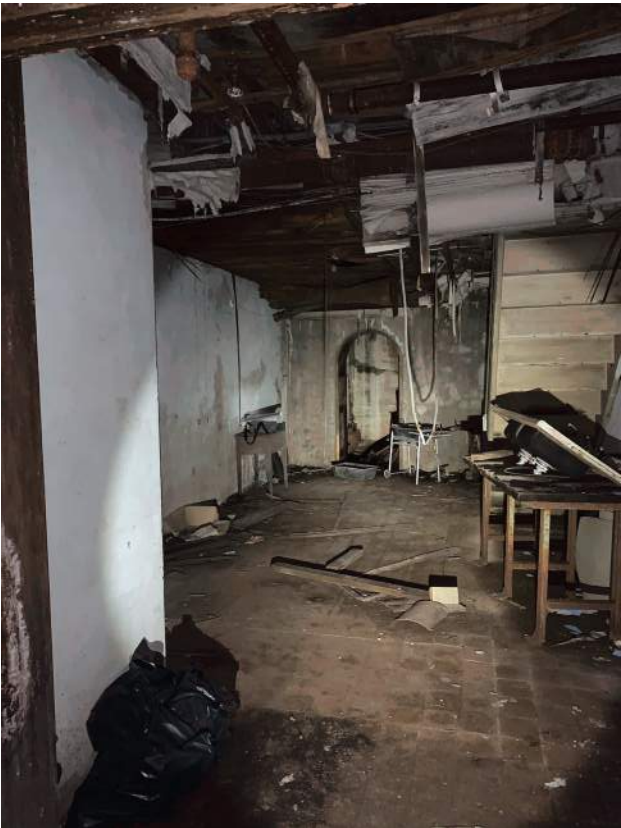
Lower Floor Level Lobby
