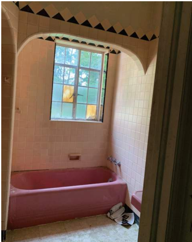
Bathtub Area of First Floor Level Bathroom
