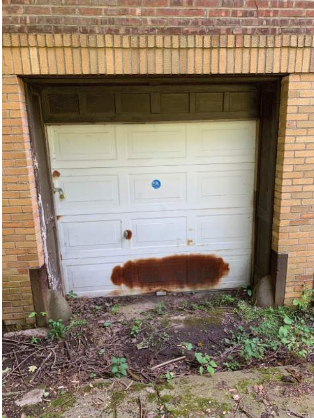
Basement Garage Door - Wood Surround
