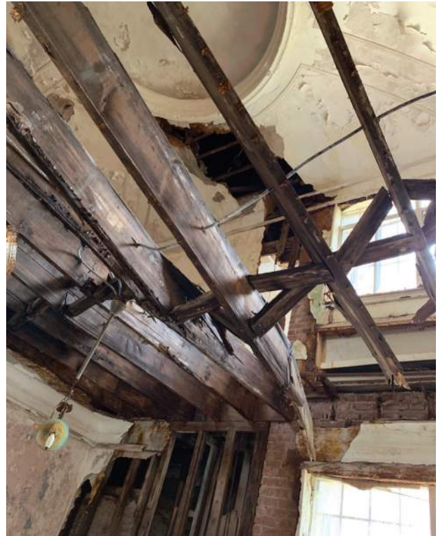
Domed Second Floor Level Reception Room Ceiling in the Background
