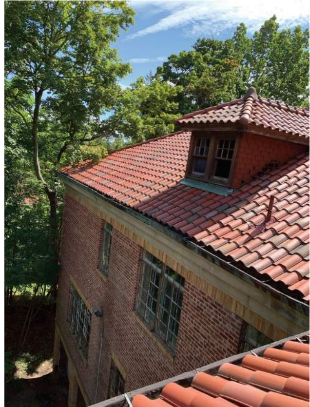
North Facing Dormer with Windows Intact
