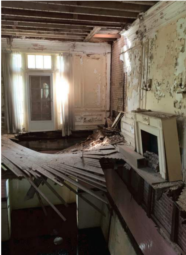
Living Room Floor and Exposed Brick at Southeast Corner
