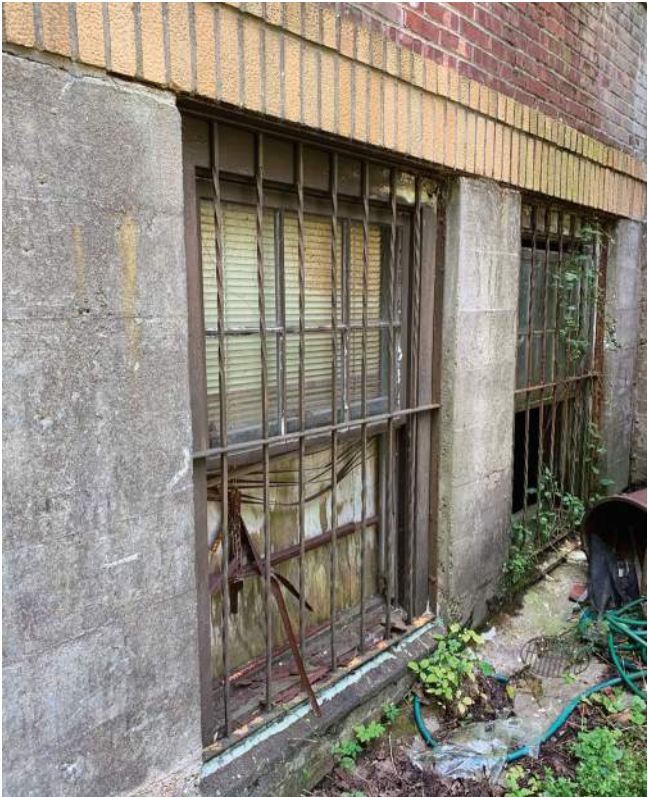
Basement Level Wood Windows
