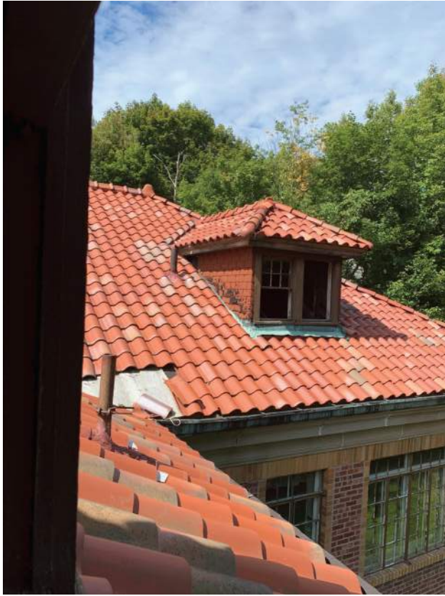
East Facing Dormer Exterior View
