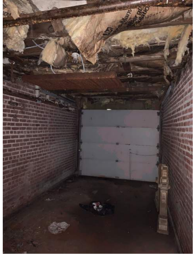
Typical Garage Condition
