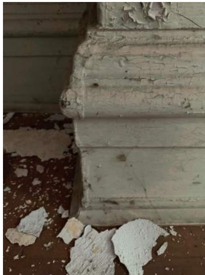
Wall Base Trim
