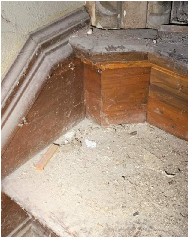
Lobby Stair Riser and Skirt Board
