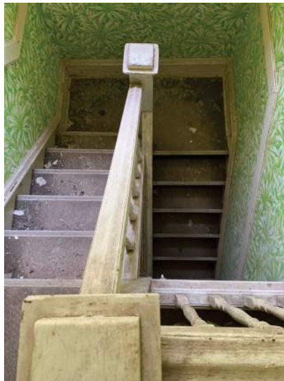
Stair Intermediate Landing
