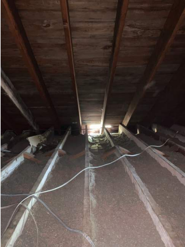
Above North Wall of Second Level Kitchen
