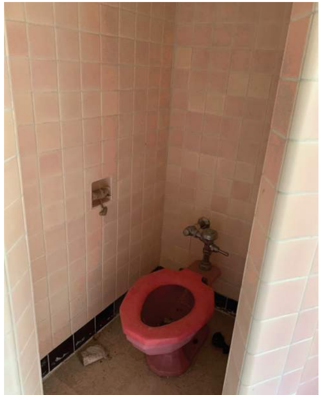
Toilet Area of First Floor Level Bathroom
