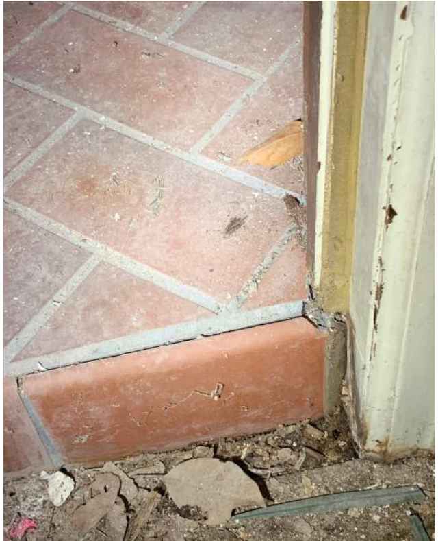
Tile and Step at Vestibule to Lobby Doorway
