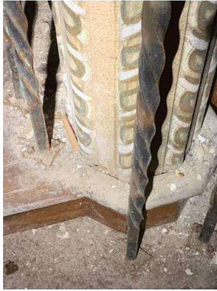
Lobby Stair Detail
