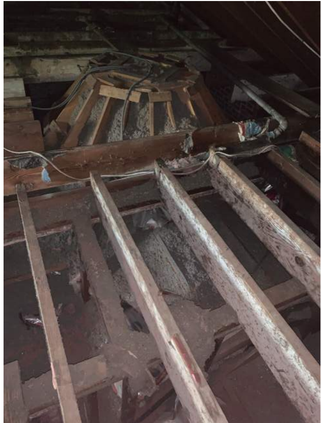
Bedroom No. 1 Framing for Bathroom Dome Ceiling
