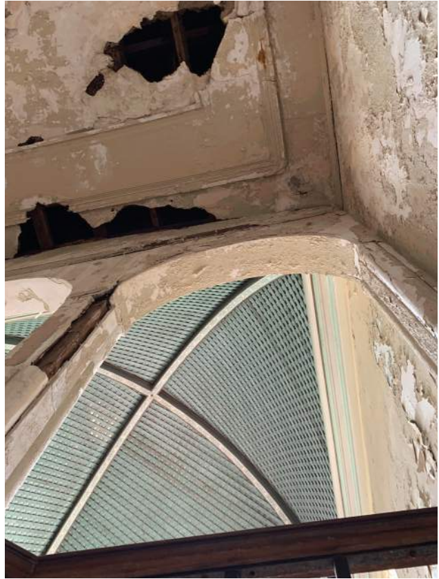
Second Level Stairhall Ceiling
