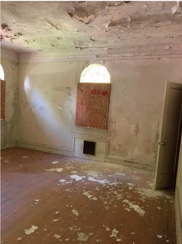
Bedroom Above Apartment Living Area, Northwest Corner of Building
