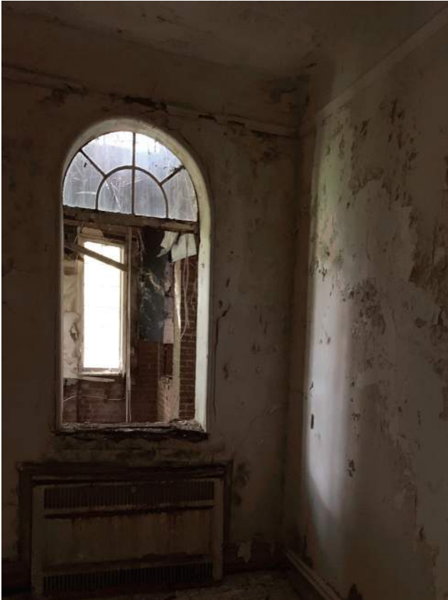
View from First Floor Level Kitchen into Southeast Sunporch
