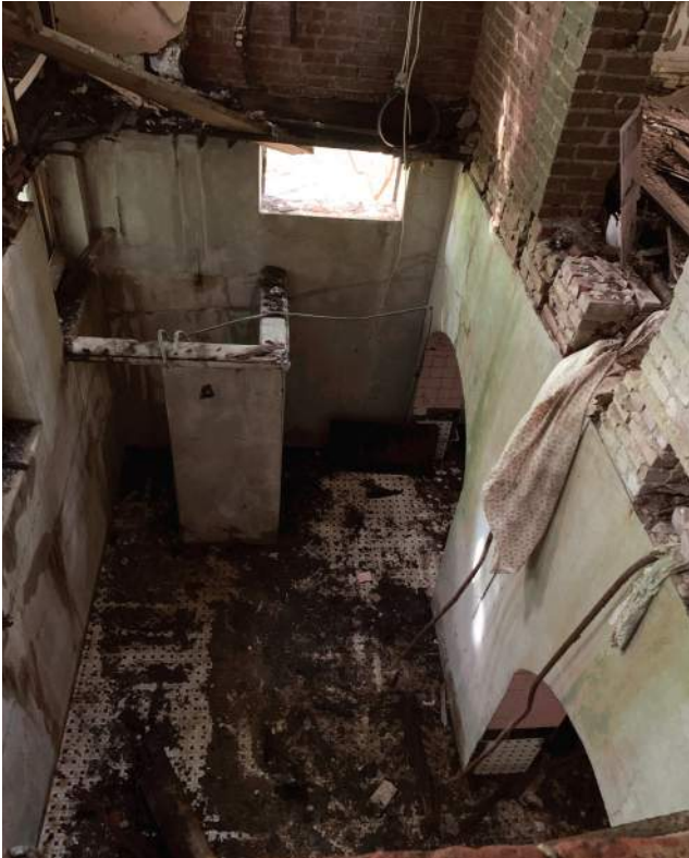
Pool Bath Beneath Southeast Sunporch
