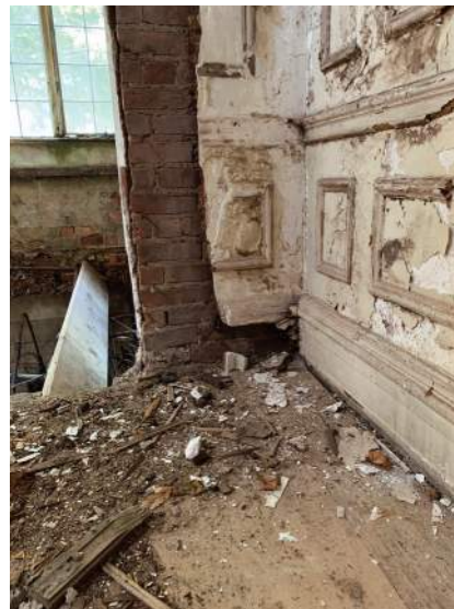
Intact Plaster Wall Panels
