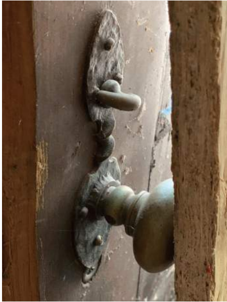
Original Hardware on Existing Front Door (Vestibule)
