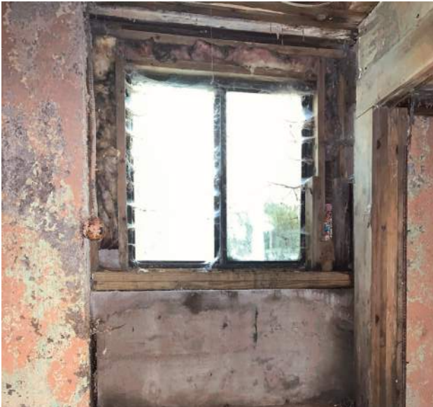
Original Lower Floor Level Window Opening Modified and Replaced
