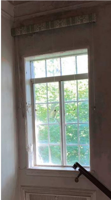
Second Floor Level Steel Casement Window with Interior Storm
