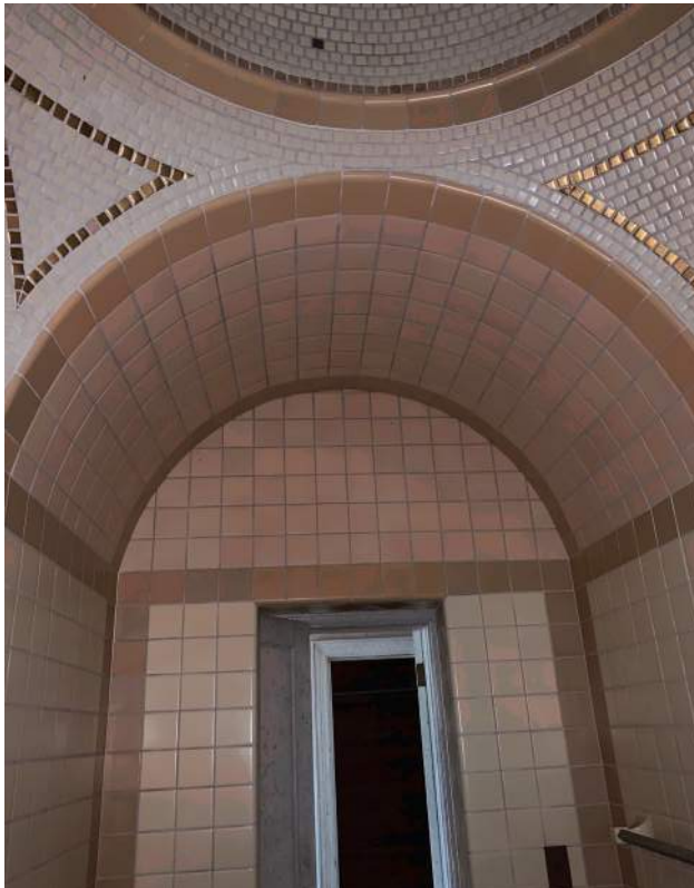
Bedroom No. 1 Bathroom Tiled Dome Ceiling Feature, Walls and Ceiling Arch
