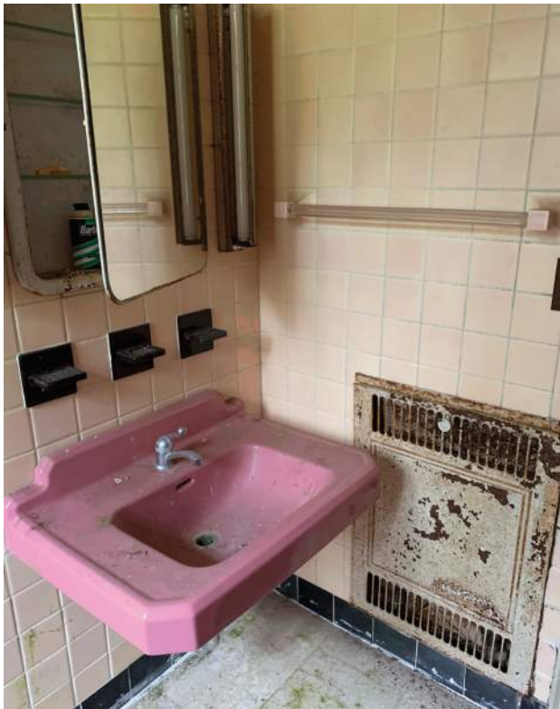
Sink Area of First Floor Level Bathroom
