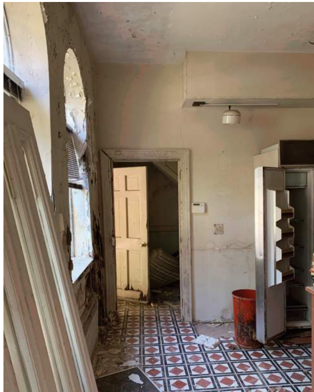
West Living Unit Kitchen
