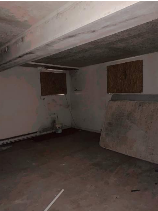
Apartment Living Area with Boarded Windows, Northwest Corner of Building
