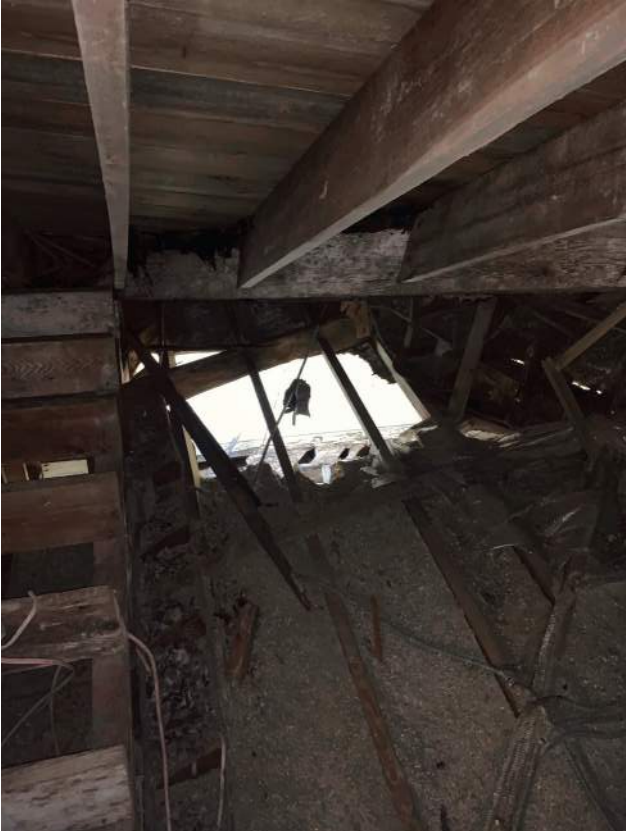
Above West Sunporch
