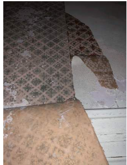
Original Wall Covering Uncovered
