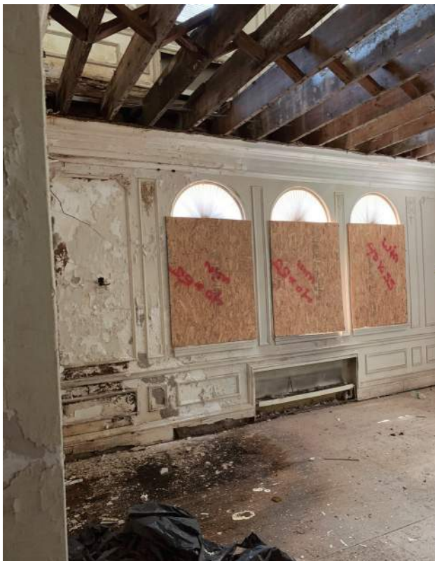
Tripartite Windows Facing Chestnut Street
