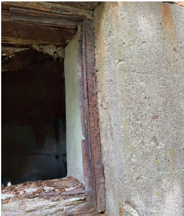
Basement Level Window Opening
