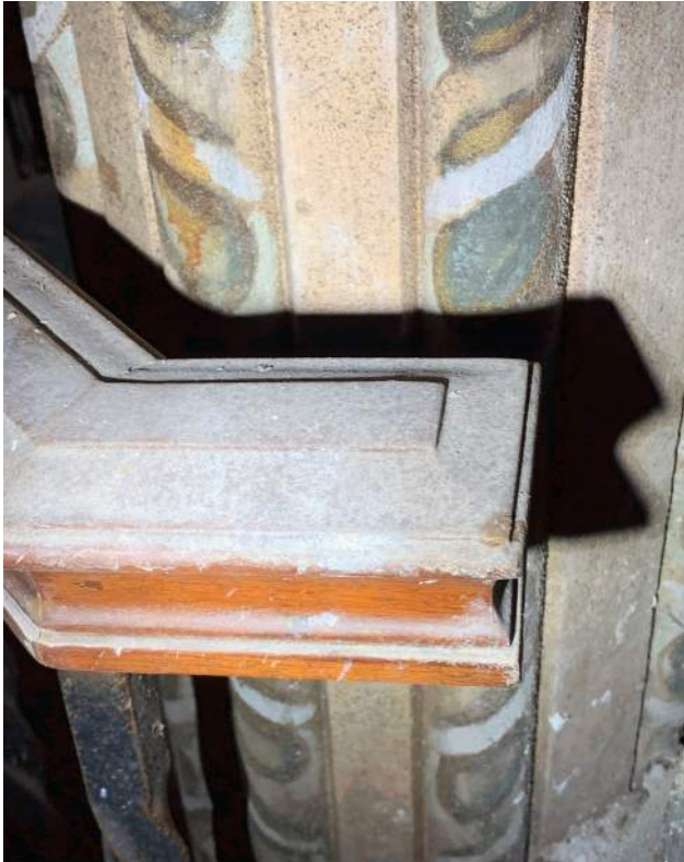
Lobby Stair Railing and Decorative Column
