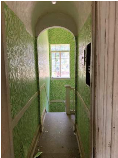
Stairhall on Second Floor Level
