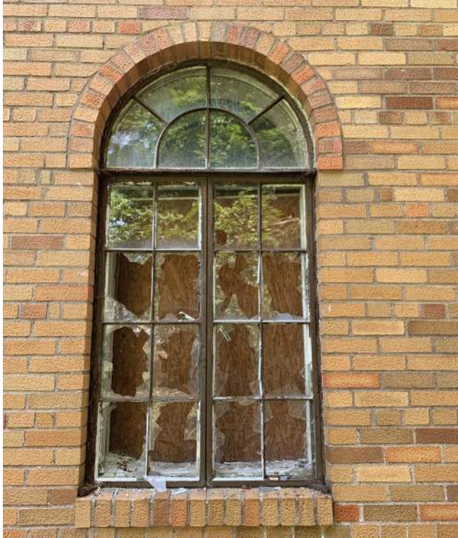
Typical Steel Casement Window with Half Round Top
