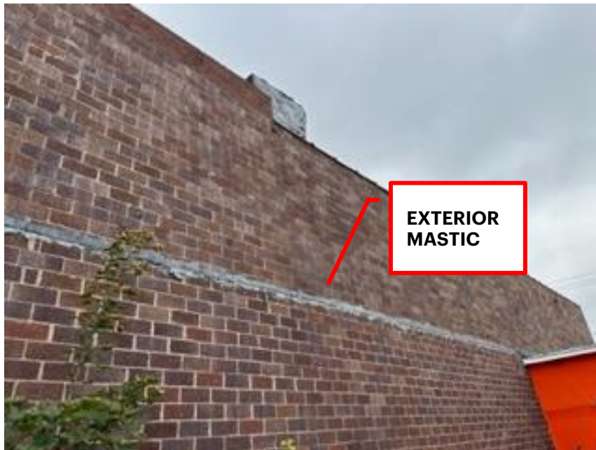
WALL MASTIC EXTERIOR
