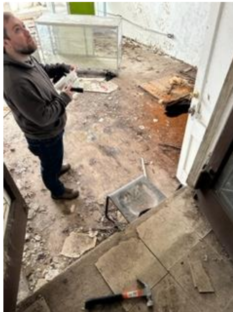
FRONT CONCESSION TILES
