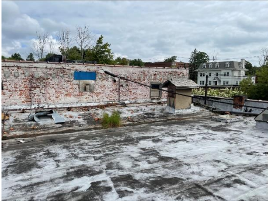
Photograph # 13 Wall to upper roof. North looking view of lower roof
