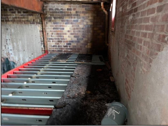
Photograph # 5 Top view of new projection room CFS floor joists.
