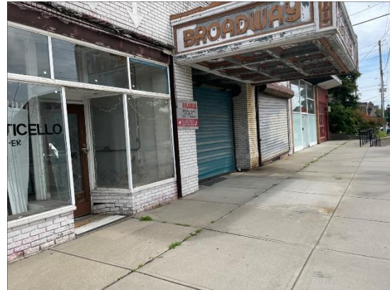
Photograph # 16 Front of building.
